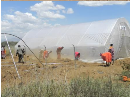
The local community helping in the erecting of the greenhouses.
